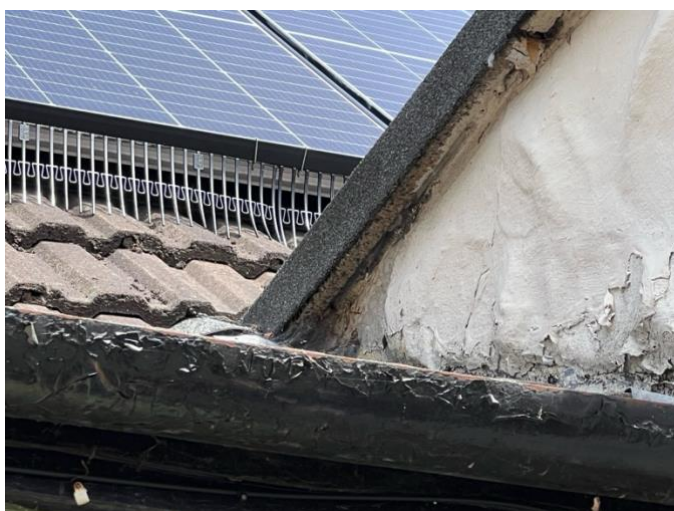
Figure 22: No access under solar panels
