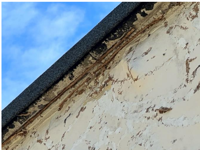
Figure 18: No access points at the wall tops or under roofing felt
