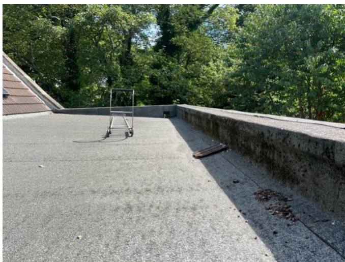
Figure 17: Flat roof on front elevation
