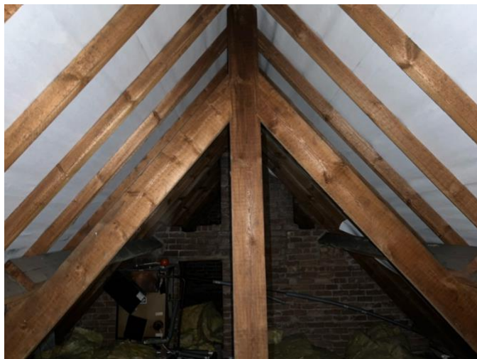
Figure 12: Attic and gable
