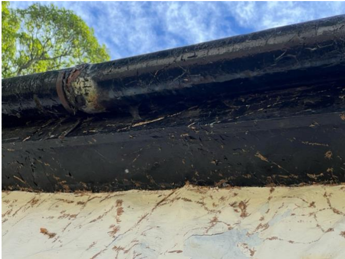
Figure 24: Guttering and metal soffit tightly sealed offering no gaps into roof space
