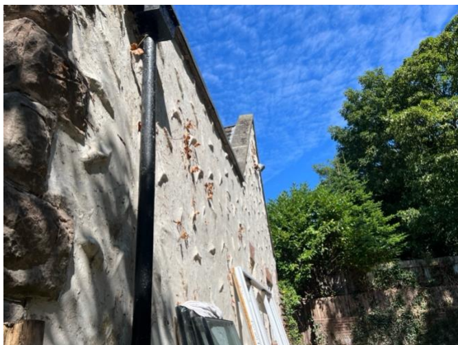
Figure 15: No gaps onto wall tops
