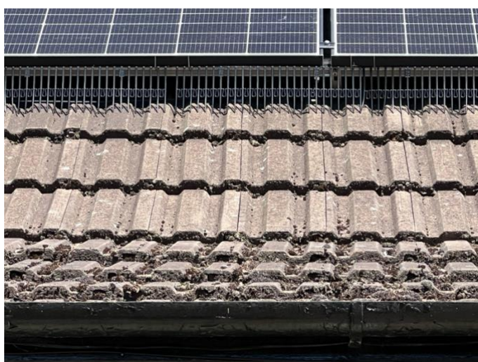
Figure 16: Tightly sealed roof tiles with no gaps
