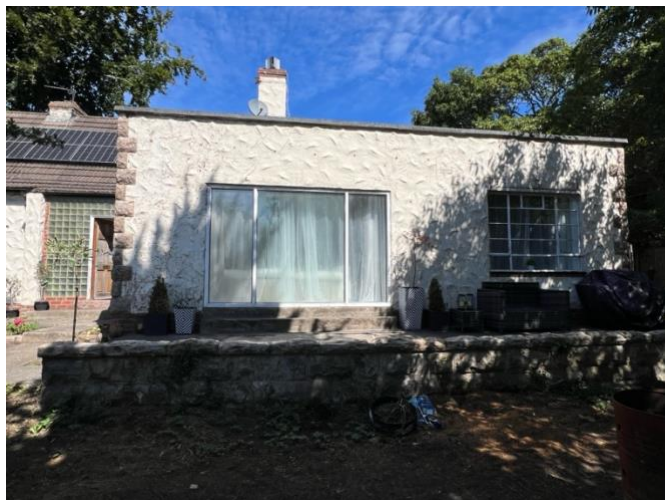
Figure 9: Flat roof section on front elevation
