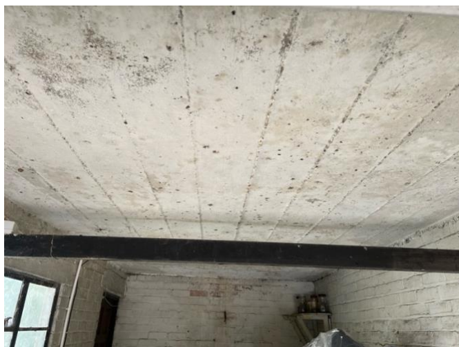
Figure 11: Interior of garage
