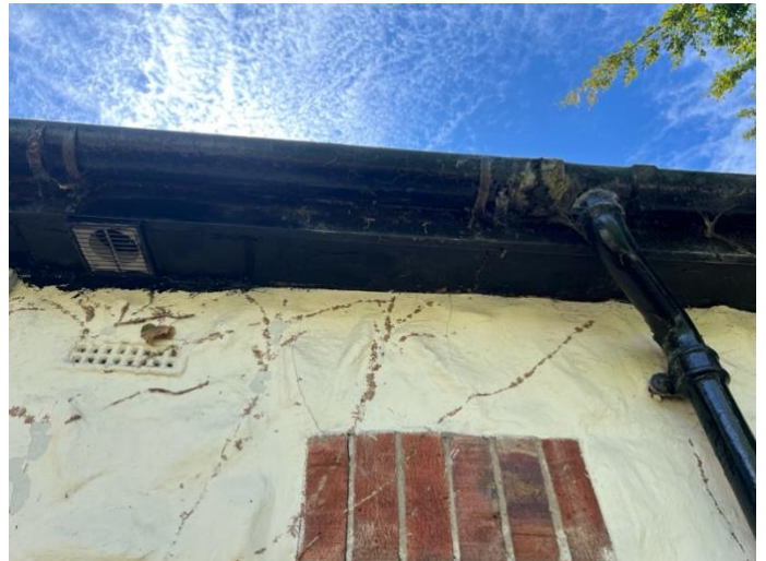
Figure 25: Guttering and metal soffit tightly sealed offering no gaps onto wall top
