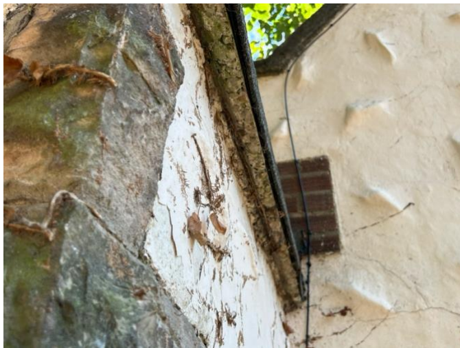
Figure 19: Tightly sealed roofing felt with no gaps
