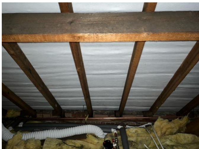
Figure 14: Plastic roof lining
